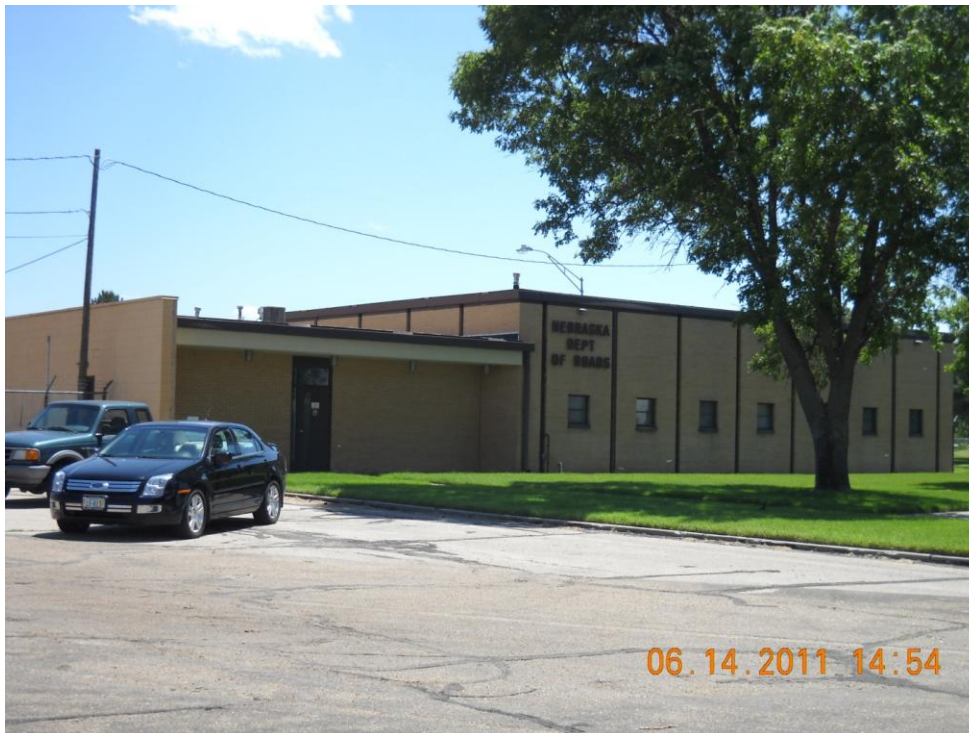
Figure 8: The Nebraska Department of Roads Maintenance yard is at elevation 2560.52 which is .6' above the 10 year flood and .5' below the 50 year flood.
