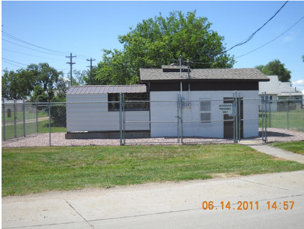
Figure 7: The municipal water well is at elevation 2558.04. It is 0.9' below the 10 year flood and 2.2' below the 50 year flood.
